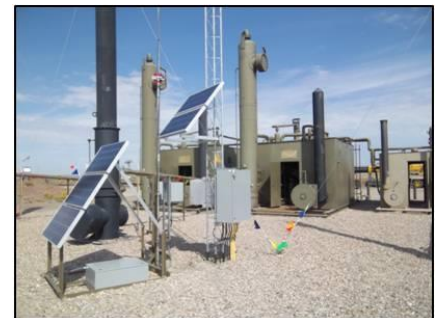
Aegis 400 placed in Class I Div 2 zone, 50' from Class I Div 1 monitoring site
