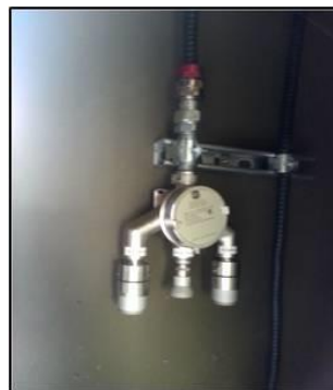
Sensors (CH 4 , H 2 S, O 2 ) located in Class I Div 1 confined space
